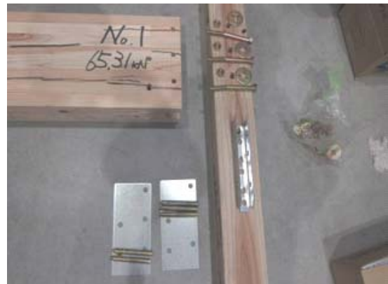
HP11-KTL007-1(カネシン)解体状況2
