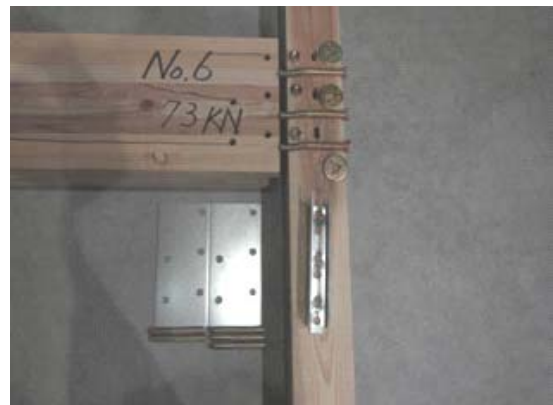
HP11-KTL007-6(カネシン)解体状況2
