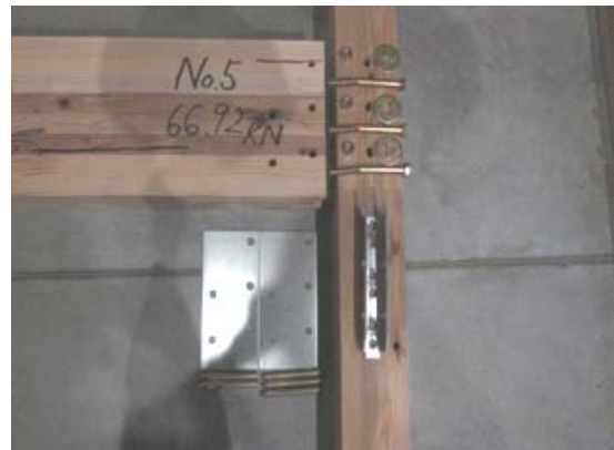
HP11-KTL007-5(カネシン)解体状況2
