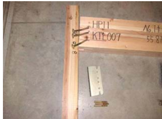
HP11-KTL007-11(タツミ)解体状況2
